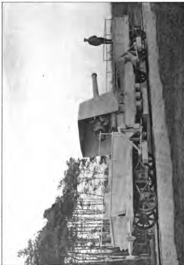
155-MM. HOWITZER (FRENCH) ON RAILWAY MOUNT.
